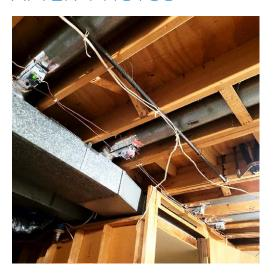
(Left) Custom zoning controls were installed in the ductwork to control the flow of air through different zones.
